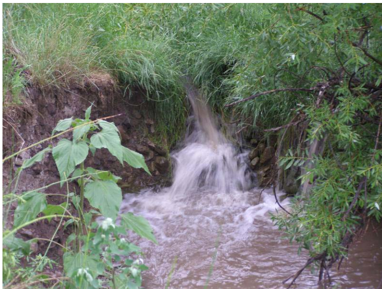
This headcut on Cedar Creek is an erosive dropoff that moves upstream, lowering the channel and the water table as it progresses.
