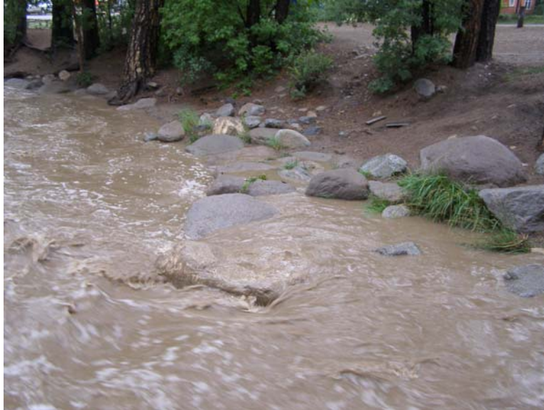
Rock vane at Two Rivers Park This protected the bank from erosion during the 2008 flood
