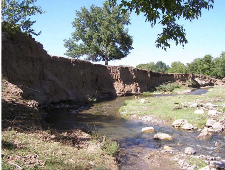
Photo taken from just below the irrigation diversion on the Stansell Ranch, looking downstream at bank erosion and scour
